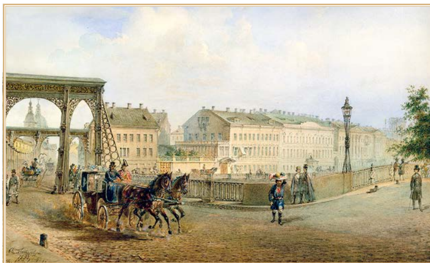
View of the Third Section building from the Chain Bridge.
